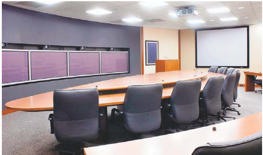
New 'telepresence' videoconferencing rooms made by Teliris feature rows of plasma television screens, as well as broadcast-quality cameras.
